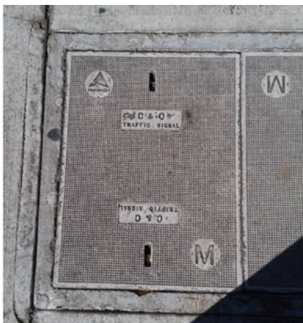
Figure 1. Manhole for Traffic Signal Cables (photo by author)
